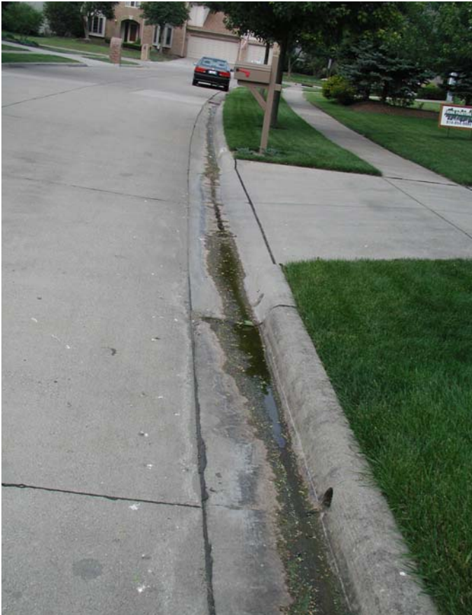
Ponding in Gutters due to uneven Concrete.
