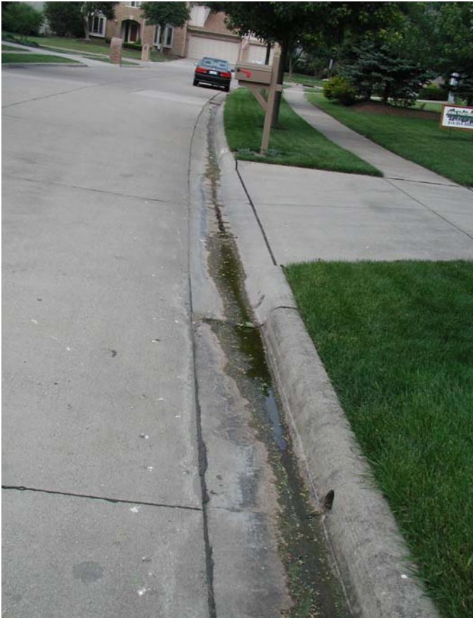
Ponding in Gutters due to uneven Concrete.
