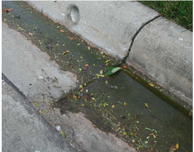
Ponding in Gutters due to uneven Concrete.
