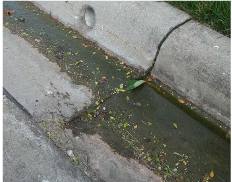
Ponding in Gutters due to uneven Concrete.
