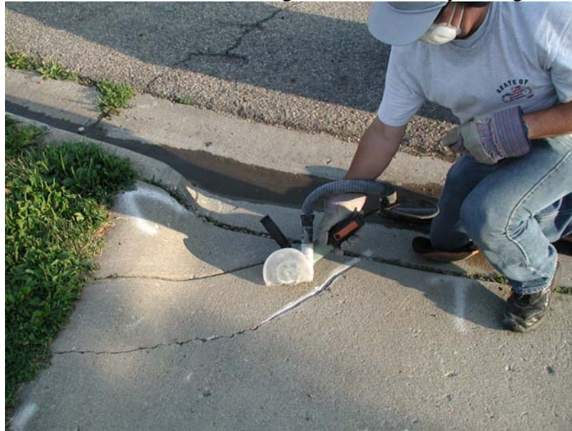
Figure 4: Midway through Crack Sealer operation.
