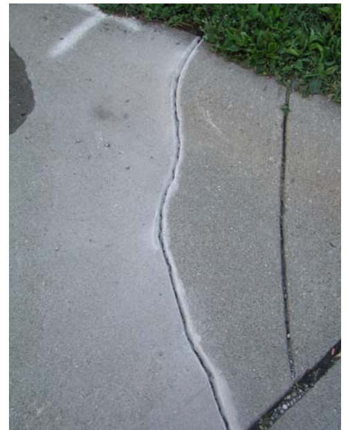
Figure 6: Finish ground Groove
