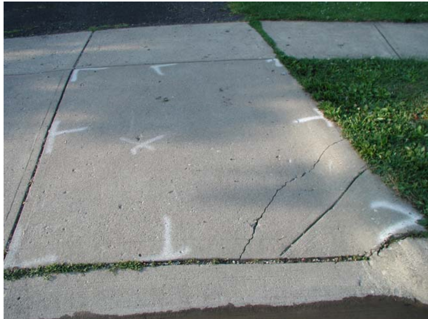
Figure 1: Driveway Apron at 7190 Anne Ct.
