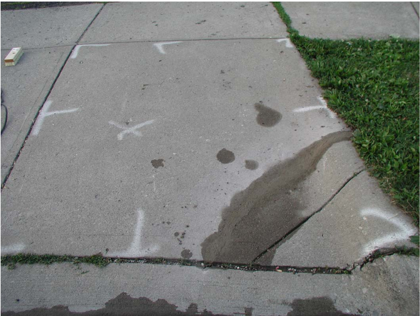
Figure 7: Final View of Patched Groove
